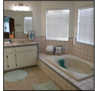
BATHROOMS Wall Conditions
