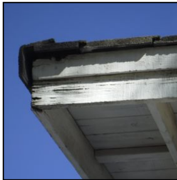
EXTERIOR AREAS Eaves & Fascia
