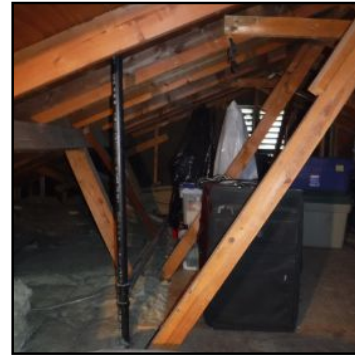
ATTIC AREA Structure
