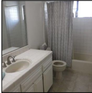
BATHROOMS Wall Conditions
