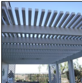
GROUNDS Patio and Porch Roofs
