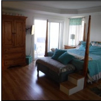
BEDROOMS Wall Conditions
