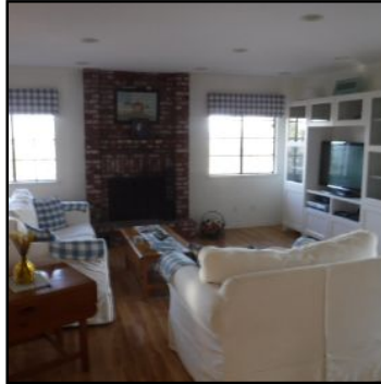
INTERIOR Wall Conditions
