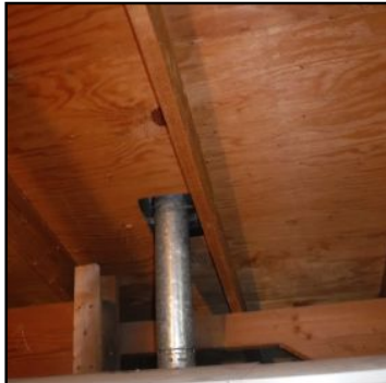
ATTIC AREA Exhaust Vents
