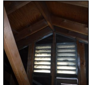
ATTIC AREA Exhaust Vents
