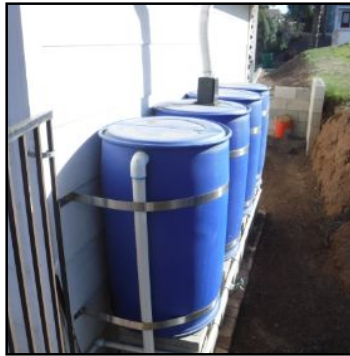
GROUNDS Exterior Plumbing and Faucets
