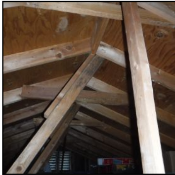
ATTIC AREA Structure
