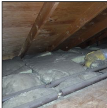
ATTIC AREA Insulation
