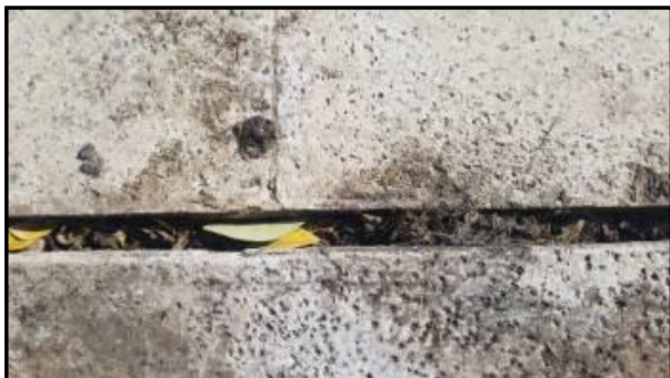
Separating from decking - Needs to be serviced
