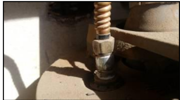
Corrosion present - signs of wear - monitor for moisture
