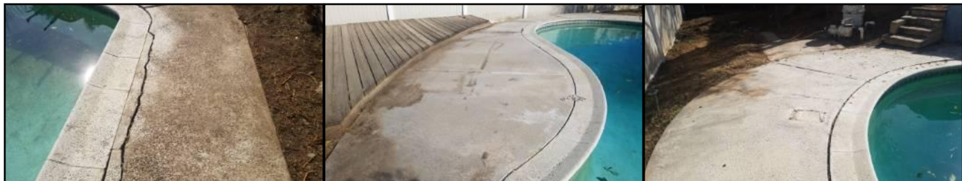
Uneven/lifted/lipage in areas – trip hazards present
