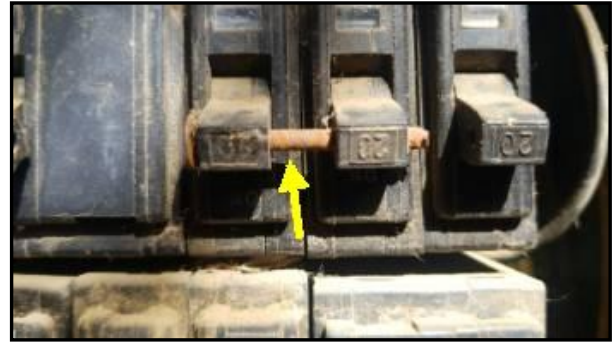
Improper breaker tie
