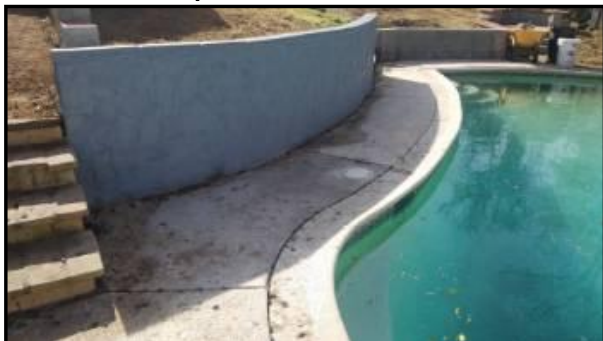
Uneven/lifted/lipage in areas – trip hazards present
