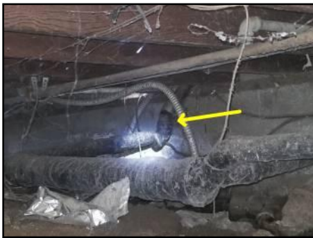
Evidence of past leakage at plumbing drain - laundry drain pipe is detached under house - ground is extremely damp in this area - needs to be serviced/further evaluation
