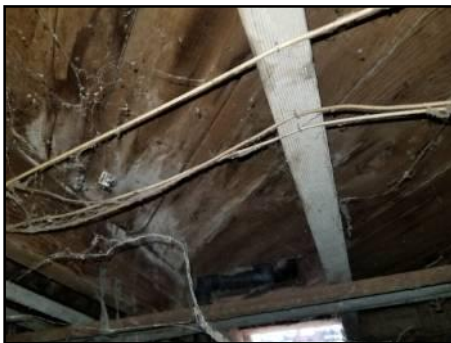
Galvanized water piping present - recommend complete water distribution system evaluation due to the age of this material
