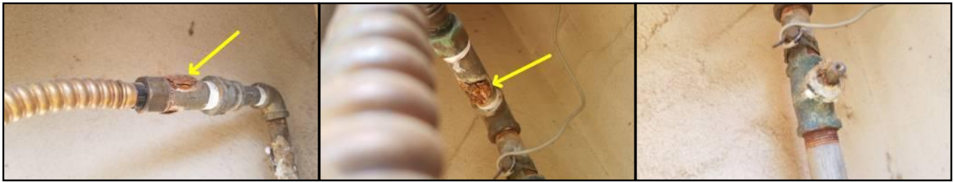
Corrosion present - signs of wear - monitor for moisture
