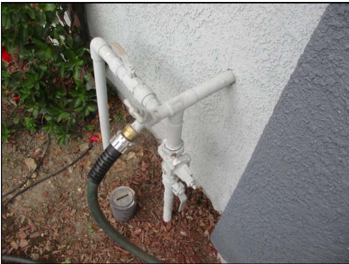
Reference Page: Grounds Reference Area: Main Water Valve
