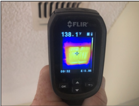
Heater Temperature at Registers:
