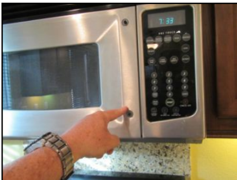
missing door handle
