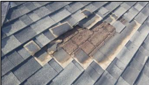
Deteriorated materials present - will require replacement at any time - consult a roofer to estimate remaining lifespan
