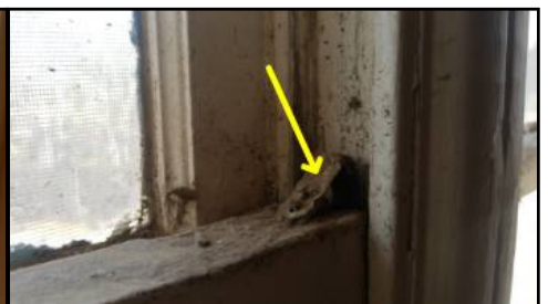
Broken sash cables or springs- unsafe - needs to be serviced
