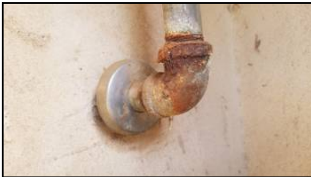
Corrosion present - signs of wear - monitor for moisture
