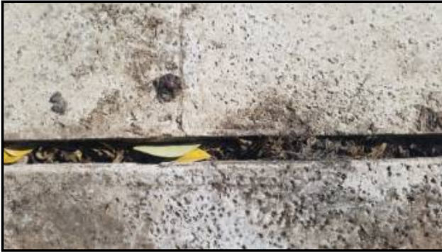
Separating from decking - Needs to be serviced
