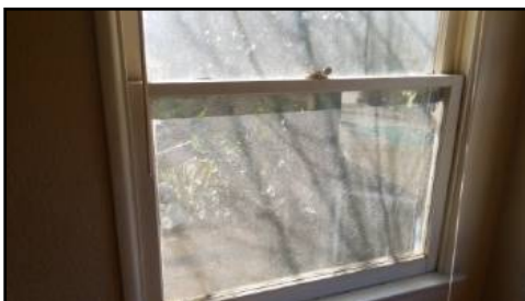
Stuck in position - needs to be serviced
