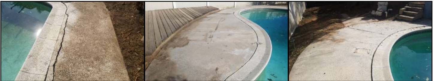
Uneven/lifted/lipage in areas – trip hazards present
