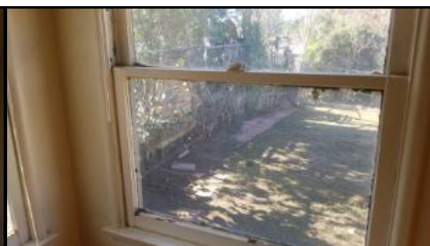
Stuck in position - needs to be serviced
