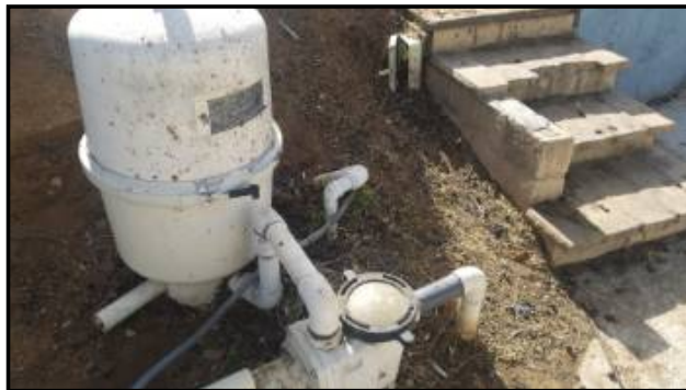
No visible outlets or GFCI - not inspected
