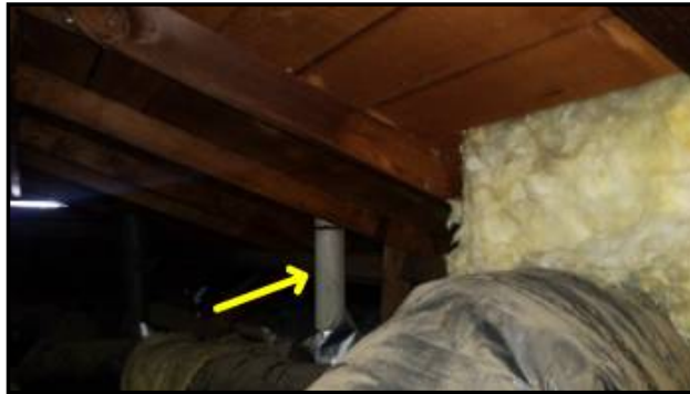
Masonry/cement/transite type vent pipe in the attic - needs to be serviced and possibly upgraded to newer style vents
