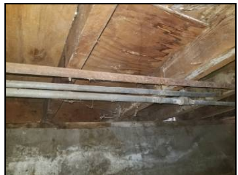
Galvanized water piping present - recommend complete water distribution system evaluation due to the age of this material
