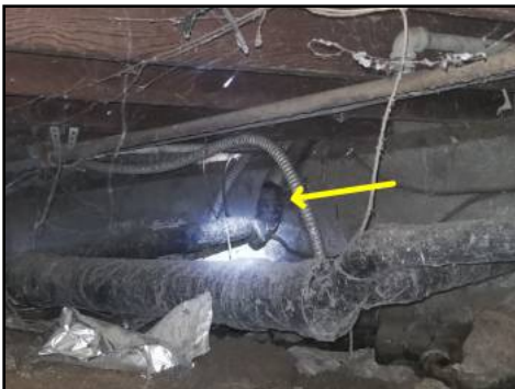
Evidence of past leakage at plumbing drain - laundry drain pipe is detached under house - ground is extremely damp in this area - needs to be serviced/further evaluation
