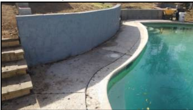
Uneven/lifted/lipage in areas – trip hazards present
